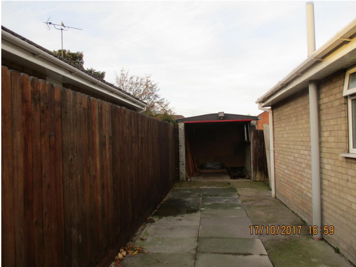
Side of application property adjacent to No. 49 Montaigne Crescent
