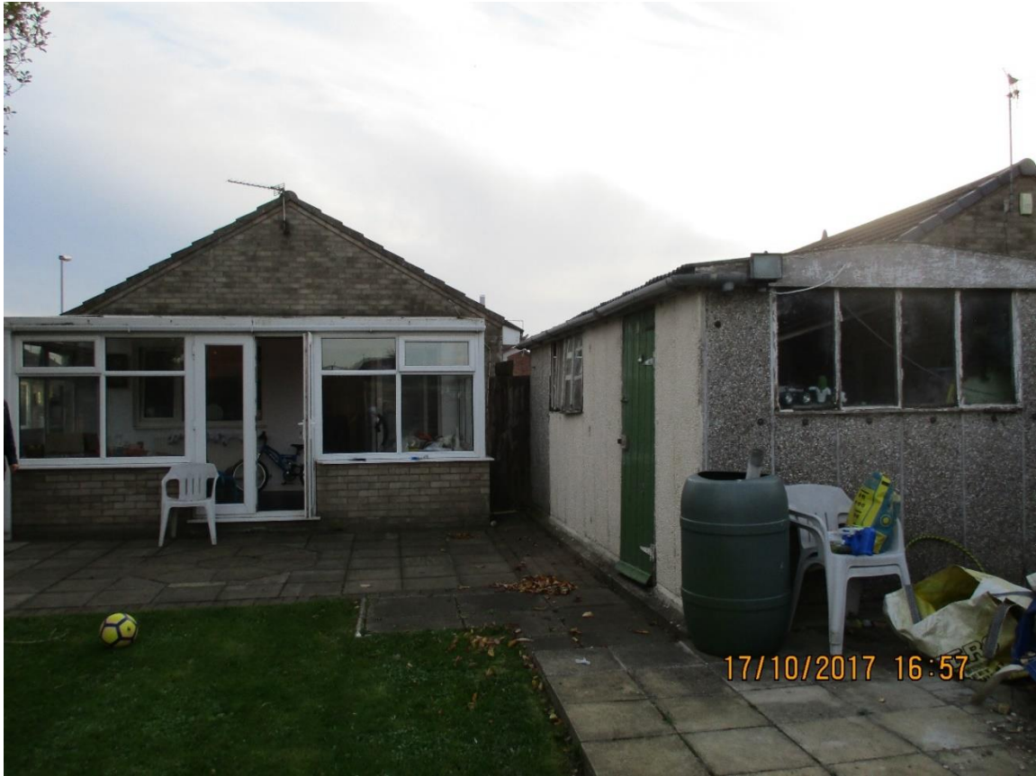
Rear elevation showing existing conservatory and garage
